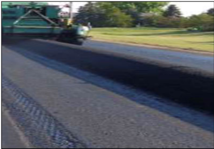
ASPHALT WINDROW EXAMPLE
